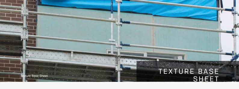
Cemintel Texture Base Sheet, commonly referred to as 'Blueboard', provides a substrate for a smooth, monolithic surface when utilising textured finishes. The products are generally used as a lightweight solution for second storey residential wraps on the ground with rendered masonry.
