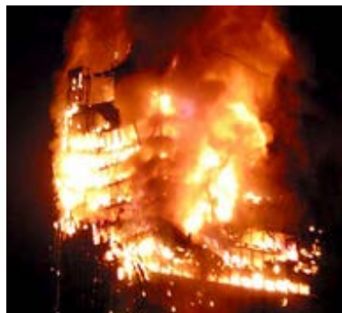
Television Cultural Centre, Beijing. February 2009. 1 person killed, 7 injured. Although illegal pyrotechnics were the cause of the fire, the 44-floor building was engulfed in about 13 mins
