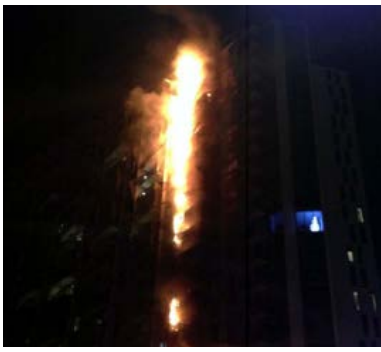
Lacrosse Apartment Fire, Melbourne. November 2014. No casualties 16 floors engulfed in about 15 mins
