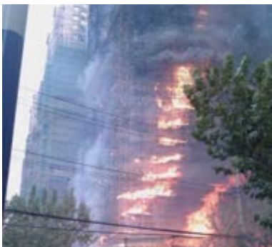
Jing An District, Shanghai. November 2010. 58 people killed, more than 70 injured. 28 storeys
