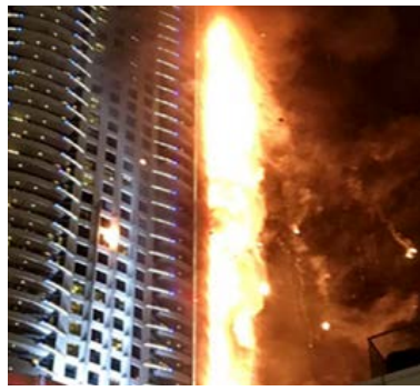
The Address Hotel, Dubai. January 2016. 14 people injured Minutes to leap 40 storeys – the cause of the fire was a short circuit
