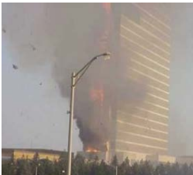
Lacrosse Apartment Fire, Melbourne. November 2014. No casualties 16 floors engulfed in about 15 mins
