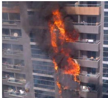
The Saif Belhasa, Dubai. October 2012. 2 injuries. 9 of the 13 storeys burnt out
